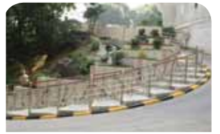
HKAH Driveway Upgraded
