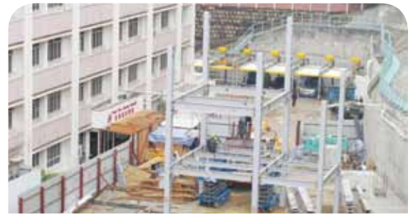
PROGRESS ON NEW WING CONSTRUCTION
