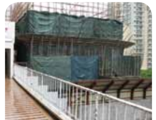
TWAH Longway Hall Demolished
